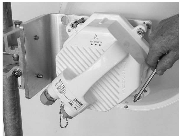
Fig. 17: Tightening bolts on the FOD unit
